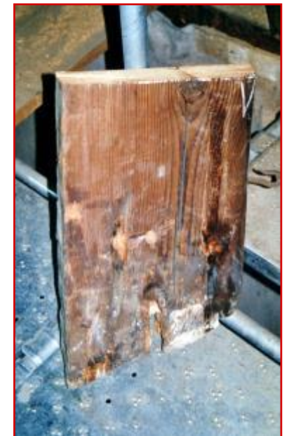
Affected top of a rib
