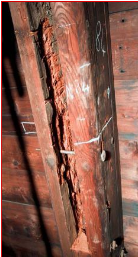
Deterioration of the internal part of a rib
