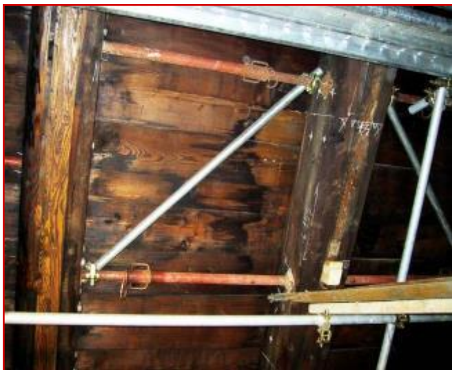
1) lateral bracing of the ribs
