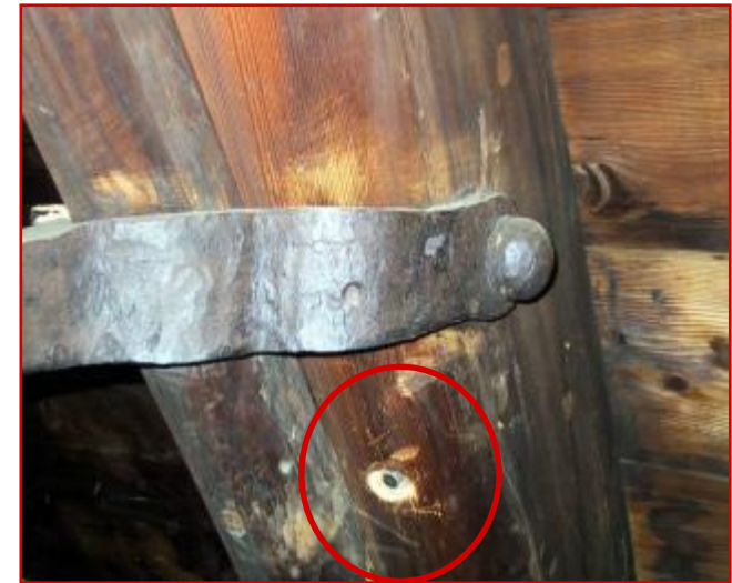
Local stitching of cracks
