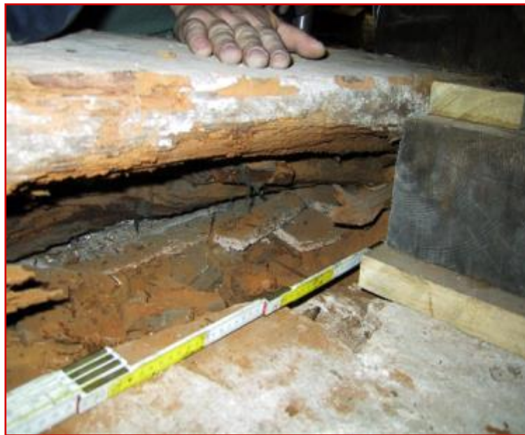
Deterioration of a shelf
