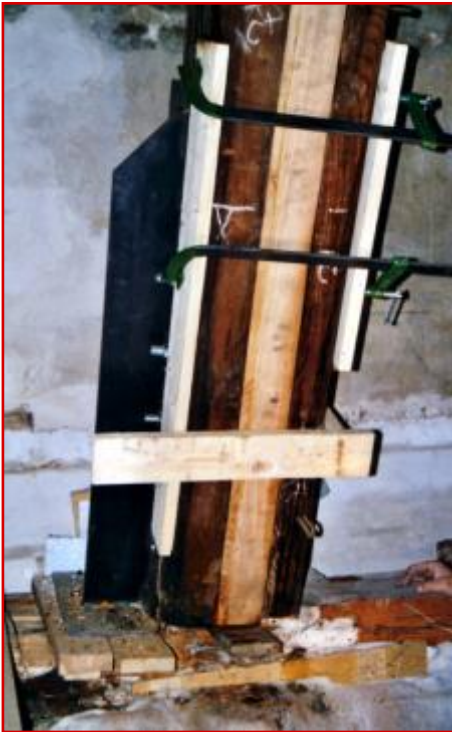
Substitution of degraded elements
