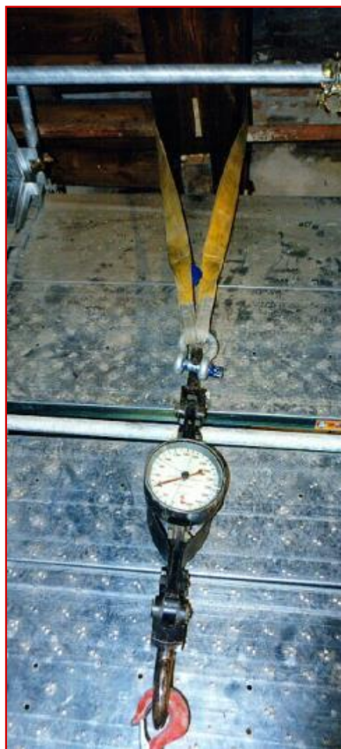
2) insertion of a temporary steel tie
